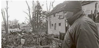
Murray Holman of Buffalo Peacekeepers surveys 79 Kilhofer St., after fire destroyed the building in 2020.
