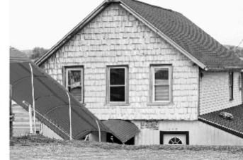
Turner's Port of Call at 997 East River Road in Grand Island is being sued by neighbors.
