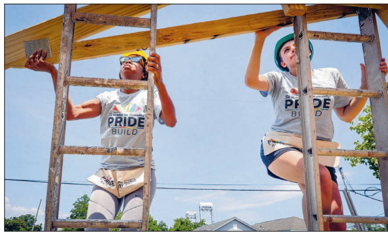
Volunteers Shaneika Dabney-Henderson and Justine Drake help raise a roof truss.
