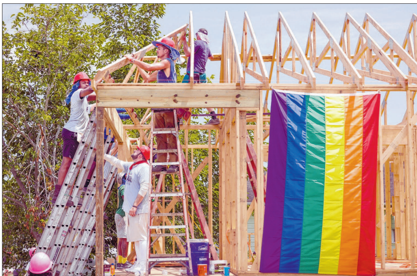
Volunteers work installing roof trusses.
